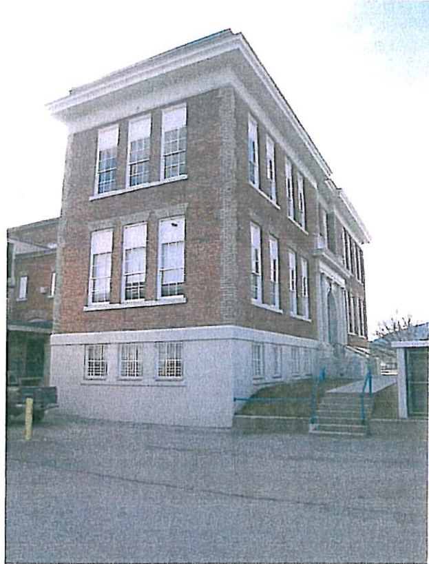
Partial east (back) elevation – March 2009 ↓
